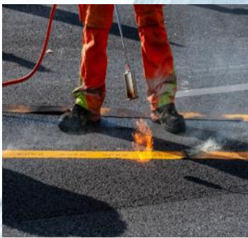
Construction Of Access Roads
