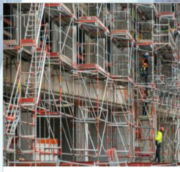
Supply And Installation Of Scaffolding System
