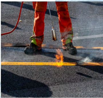
Construction Of Access Roads
