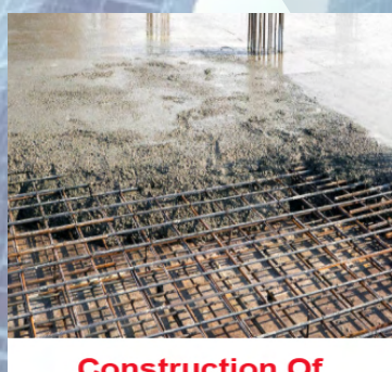
Construction Of Reinforced Cement Concrete
